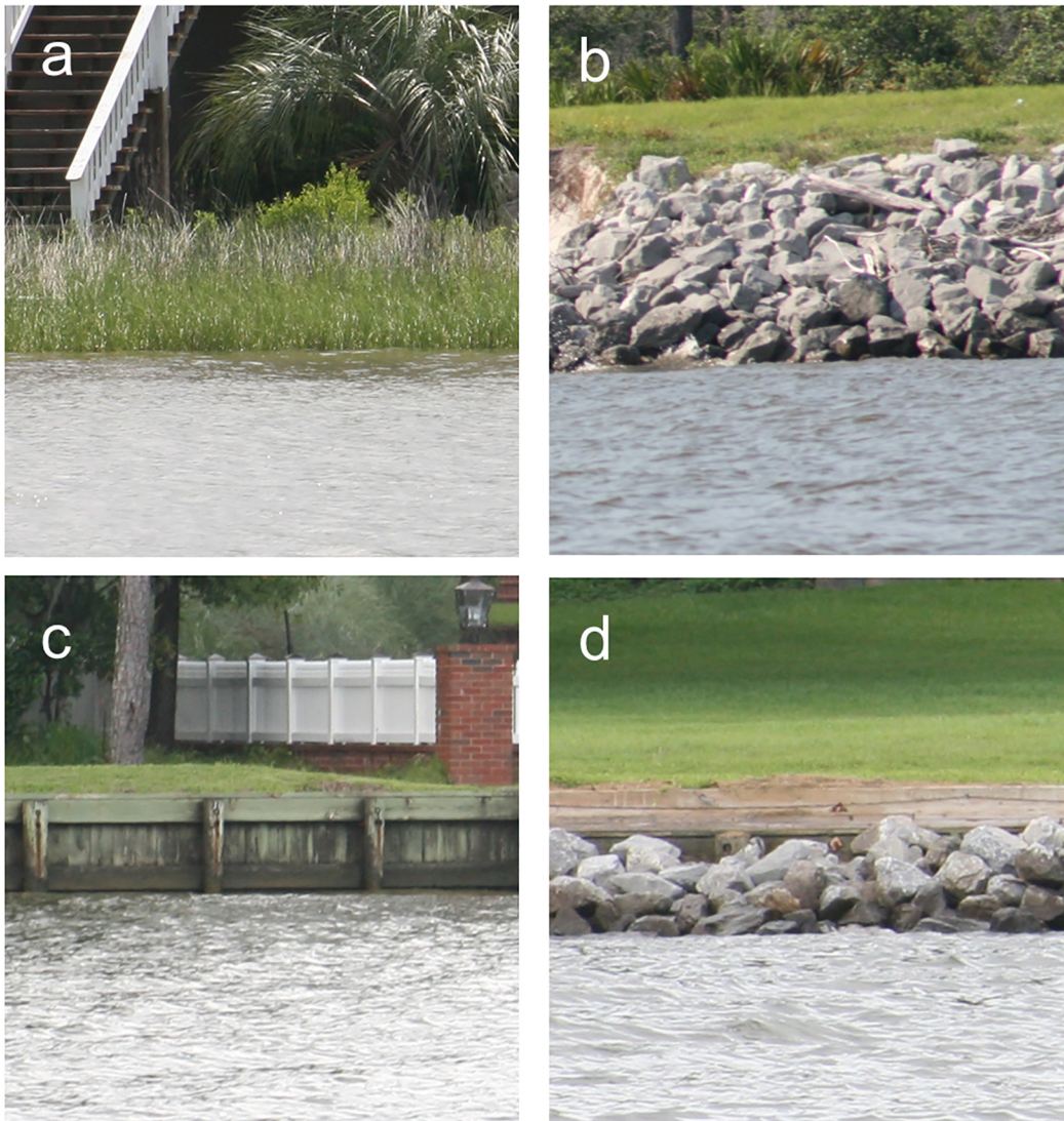
Fig 1. Example photographs of shoreline types. Photographs of (a) natural, (b) riprap / rubble, (c) vertical wall and (d) vertical wall with riprap shorelines in the study system.
