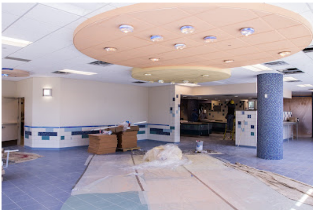
The expansion features a new dining area that is four times larger than the current cafeteria. The new dining area, which seats up to 140 people, is available for hospital visitors and staff.
